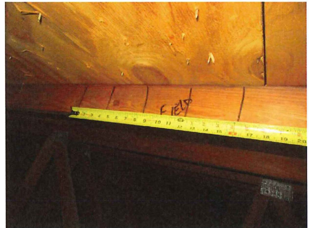
Roof Deck Nail Spacing - Field
