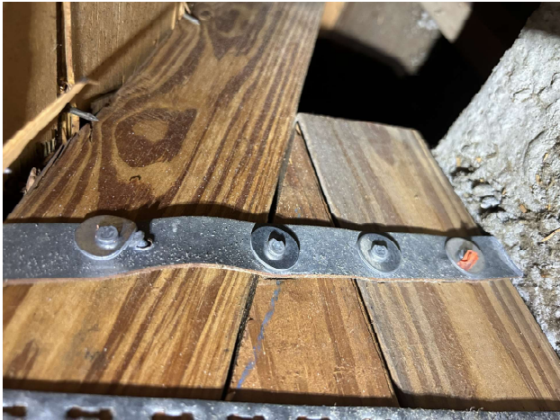
Roof to wall attachment - Clips
