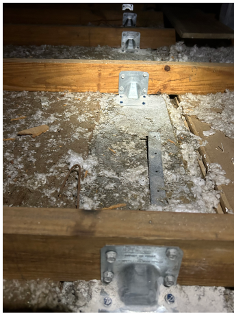
Roof to Wall - Clips
