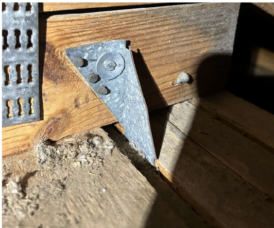
Roof to wall attachment - Clips
