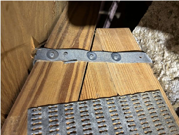
Roof to wall attachment - Clips
