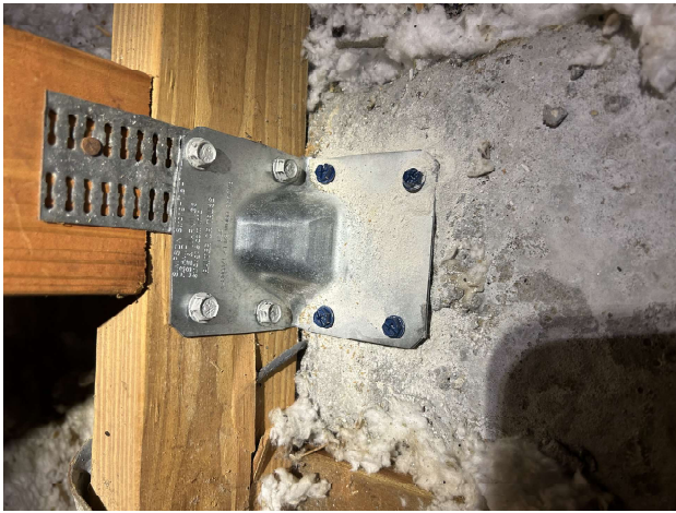
Roof to wall attachment - Clips
