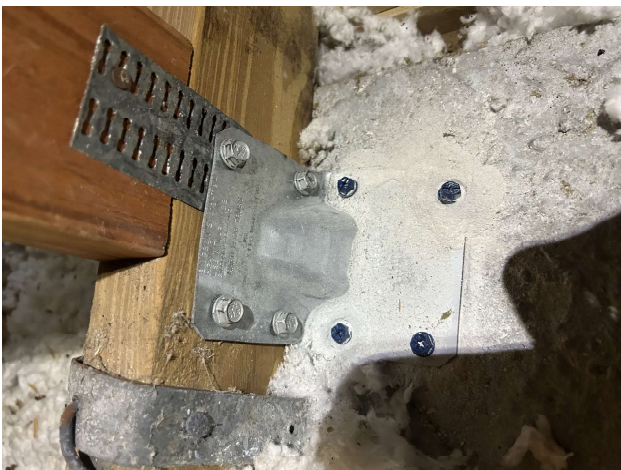
Roof to wall attachment - Clips
